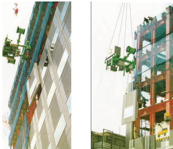
Fig. 12. Mechanizing the position of a wall element by special equipment.
