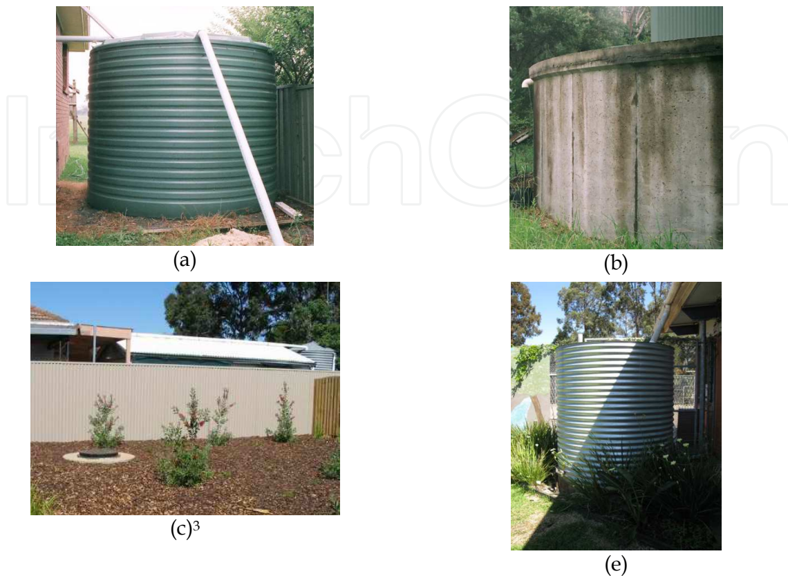
Fig. 2. Rainwater tank site locations and materials
