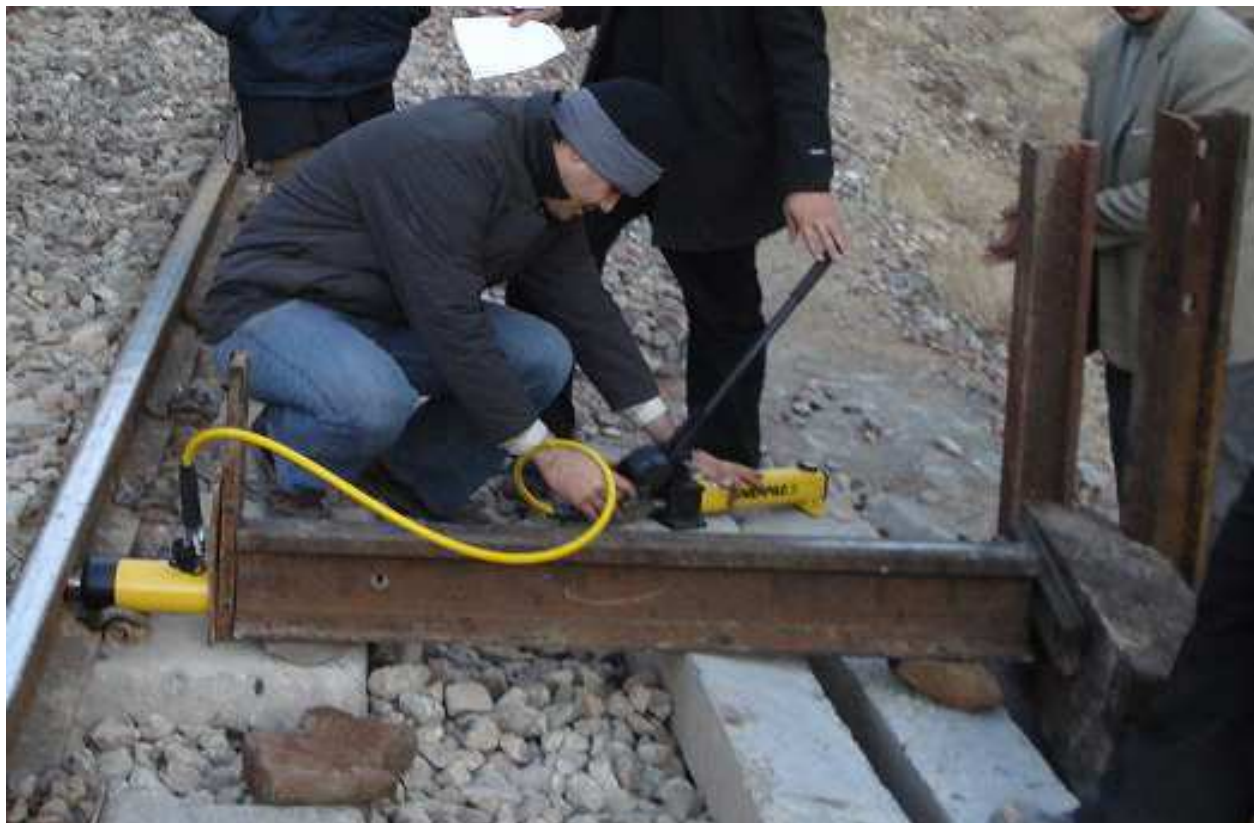
Fig. 15. Installation of the hydraulic jack
