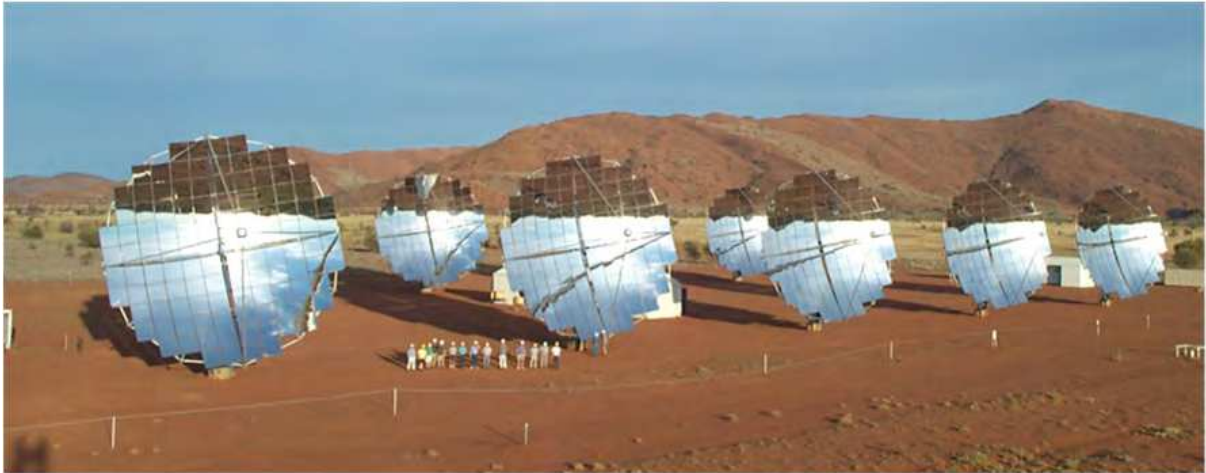
Fig. 3. Several 25-kW CPV systems built by Solar Systems in Hawthorn, Australia, and installed on aboriginal land. These systems use mirrors for concentrating sunlight onto silicon solar cells---see www.solarsystems.com.au The people in the foreground give an idea of the system's size (photo by R. McConnell).
