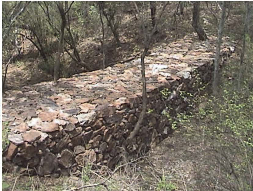
Fig. 3. Retenidas for runoff control in La Labor
