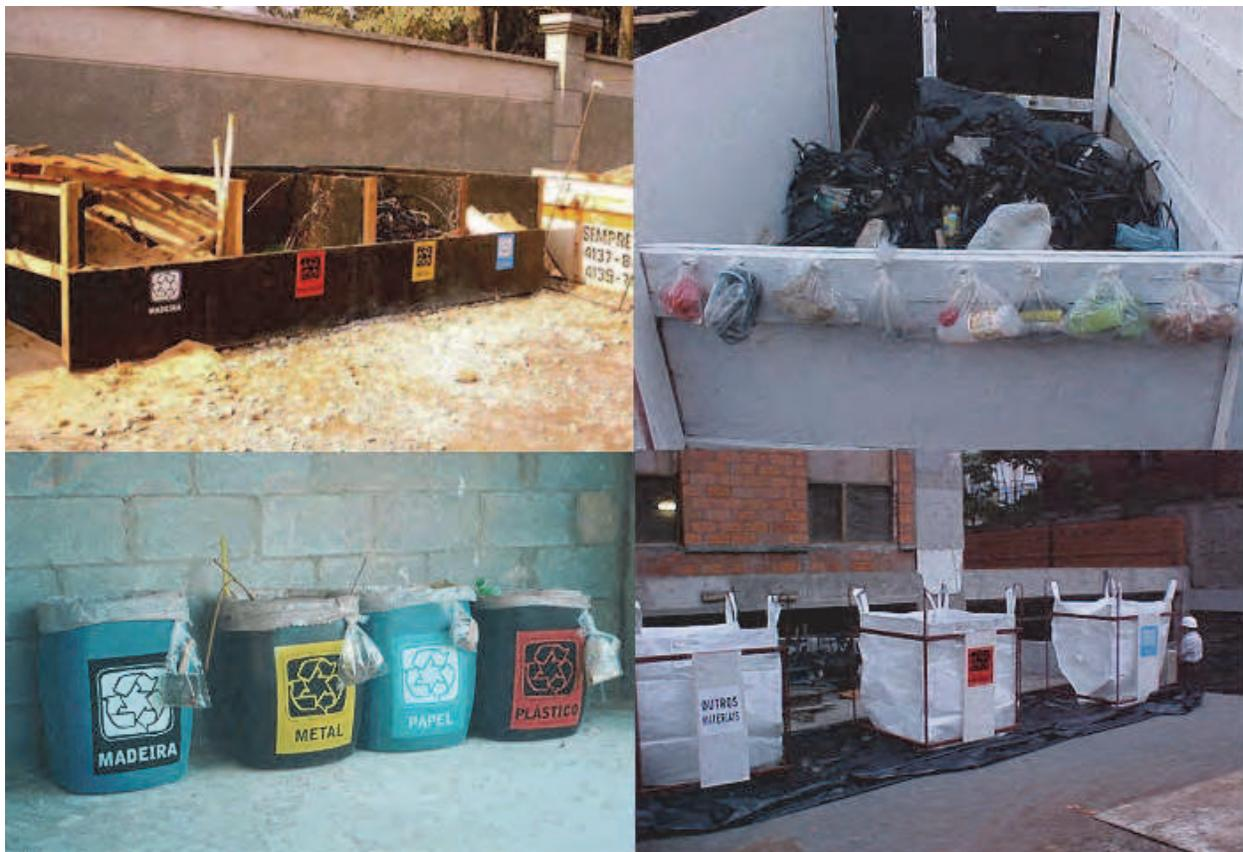
Fig. 4. Segregation of waste at the construction site
