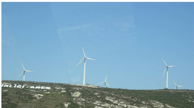
Fig. 8. A wind power plant in Çeşme-Alaçati
