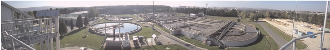
Figure 3. Zalaegerszeg wastewater treatment plant with biomethane filling station. Source: Own photo.
