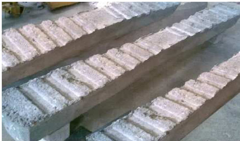
Fig. 14. The bottom of frictional concrete sleeper
