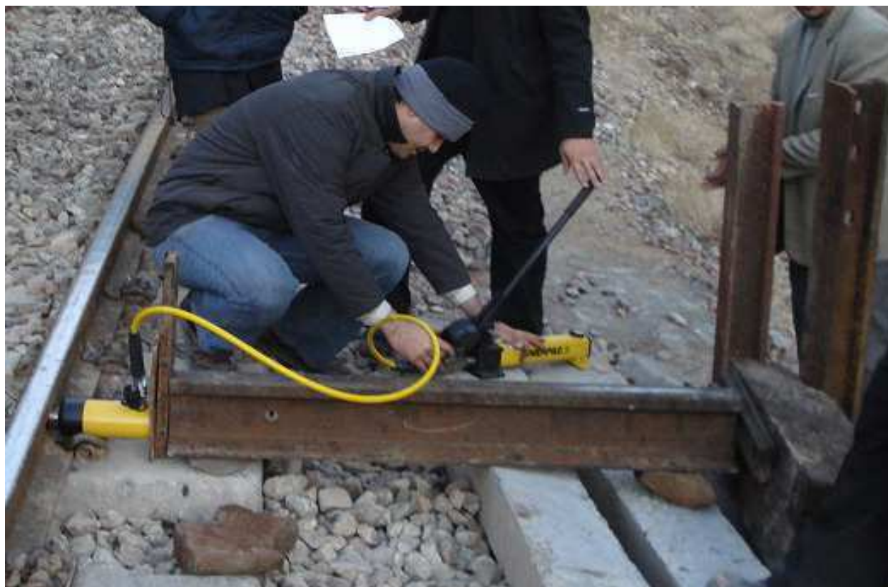
Fig. 15. Installation of the hydraulic jack
