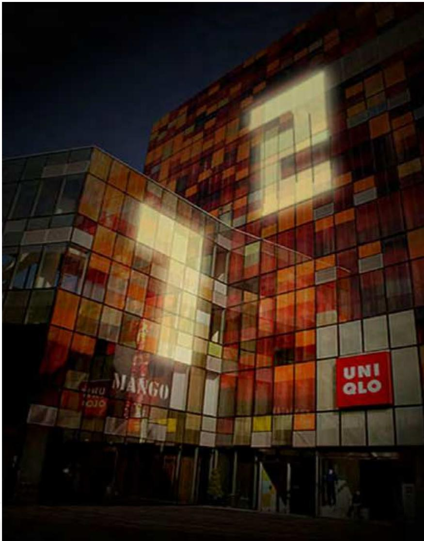
Fig. 10. FEEL can be applied to building skylights and building elevation windows. The building elevation looks like a large size display when every FEEL glass is independently controlled the turn-on status.
