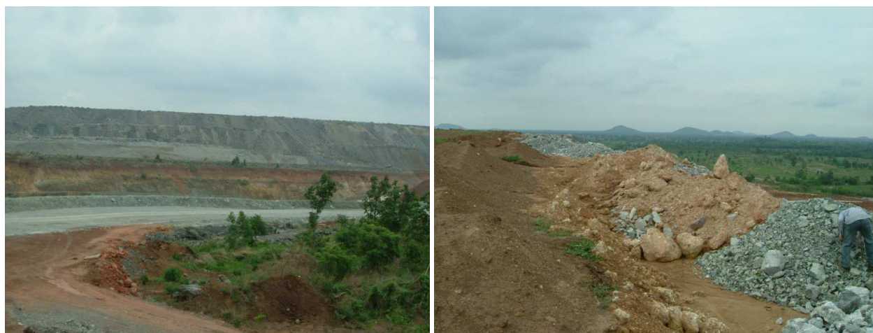
Fig. 1. Huge amount of rock waste generated from a gold mine in Thailand: left photo is waste dumping site; right photo shows placing process based on geochemical properties of each type of waste rock
