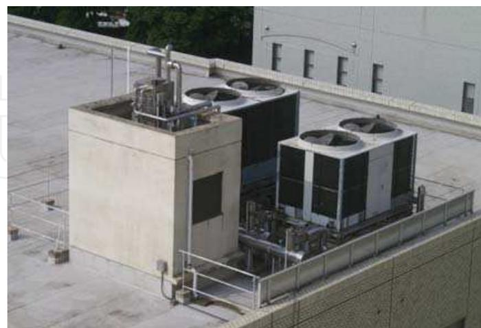
Fig. 14. Heat pump - chiller units
