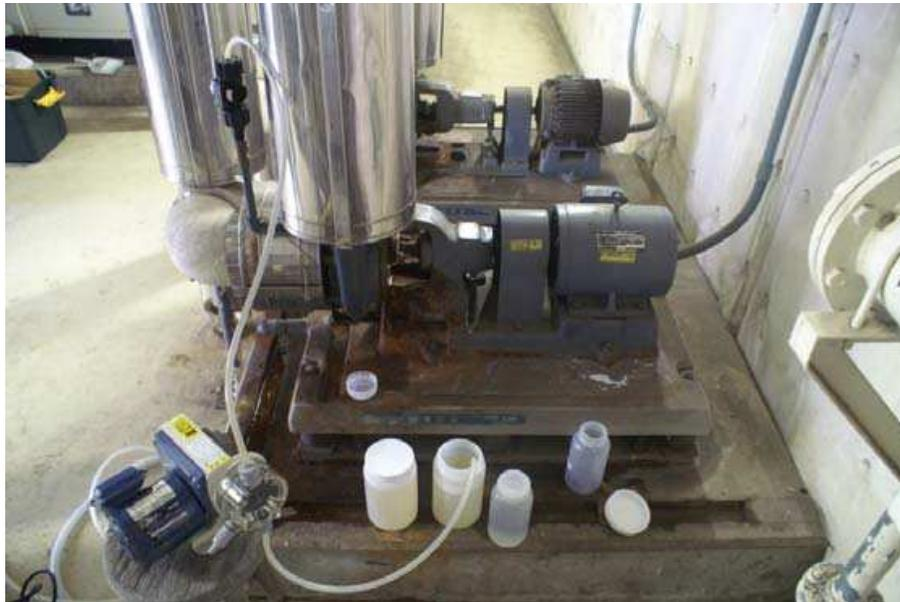
Fig. 16. Addition of LSP-01 from the discharged side of the main pump
