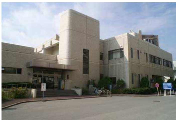
Fig. 13. Yamaguchi University library building
