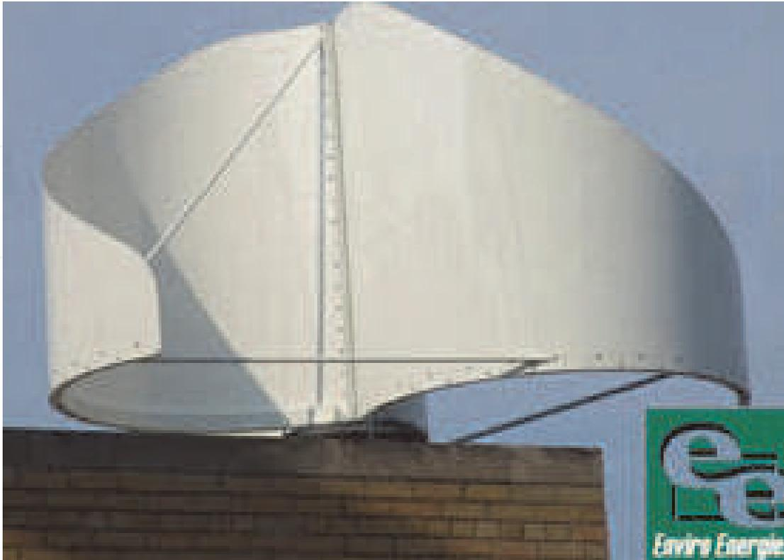
Fig. 2. VAWT made by Enviro-Energies and installed on the company's roof
