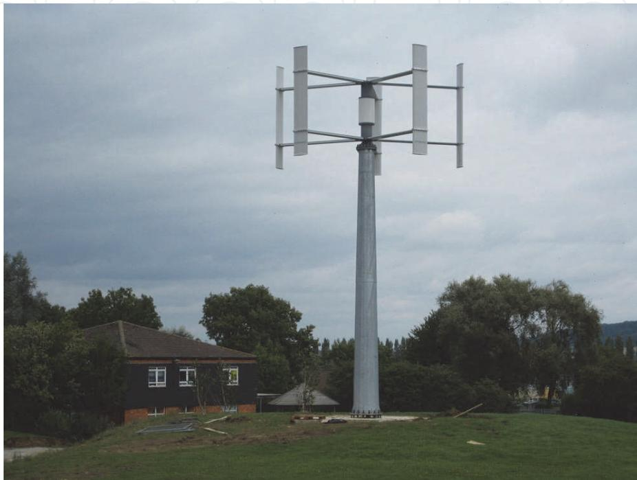
Fig. 4. H-type VAWT made by Ropatec of Italy
